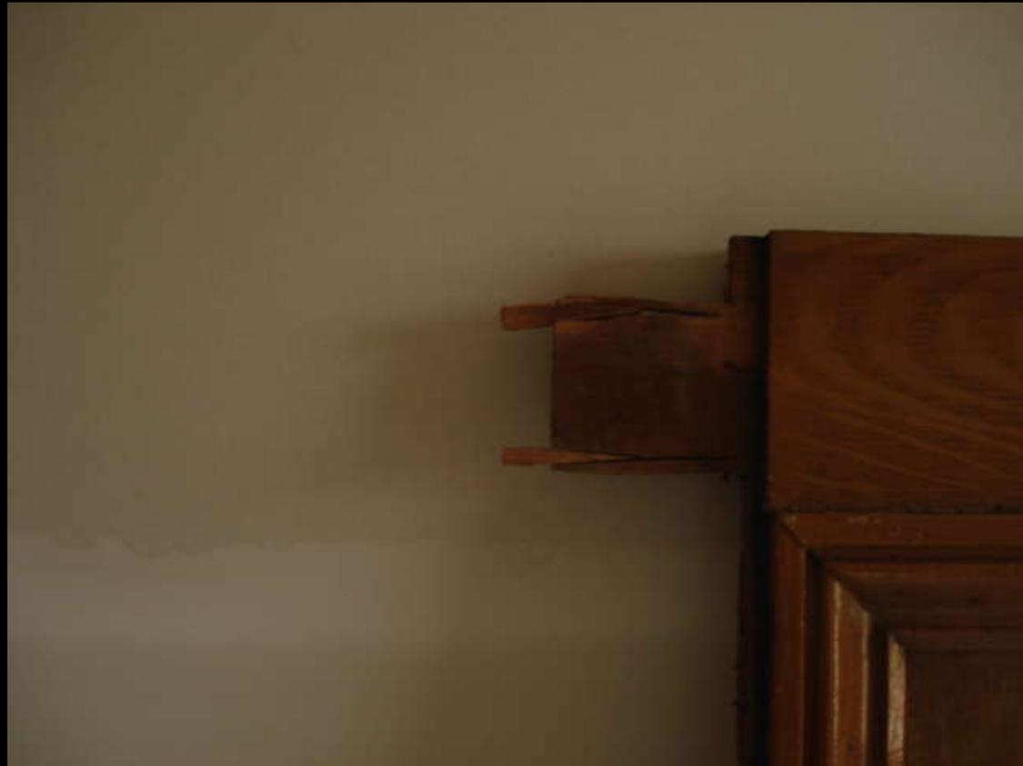
**The tongue was split top & bottom and wedges driven in to tighten – and no glue was used – and it held since 1860!**
