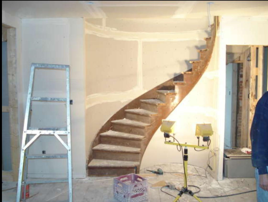
**In 1860 the carpenter trimmed the back of this side panel with an adze**
